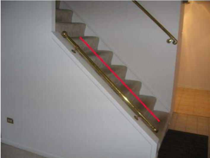
Improper handrail
