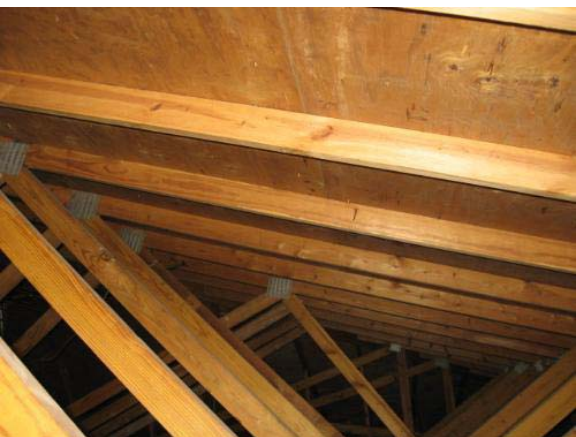
View of roof structure
