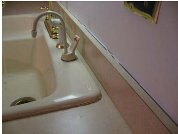
Caulk counter backsplash
