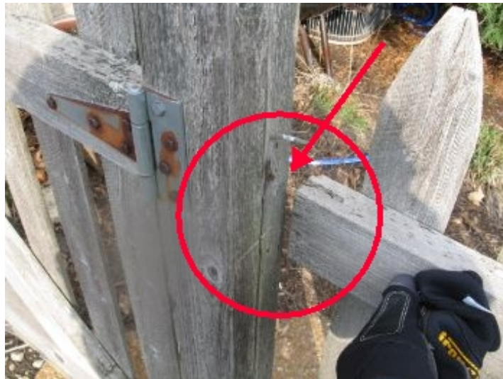
Wood fence is weathered with areas of loose fencing and sagging fence posts; repair as needed
