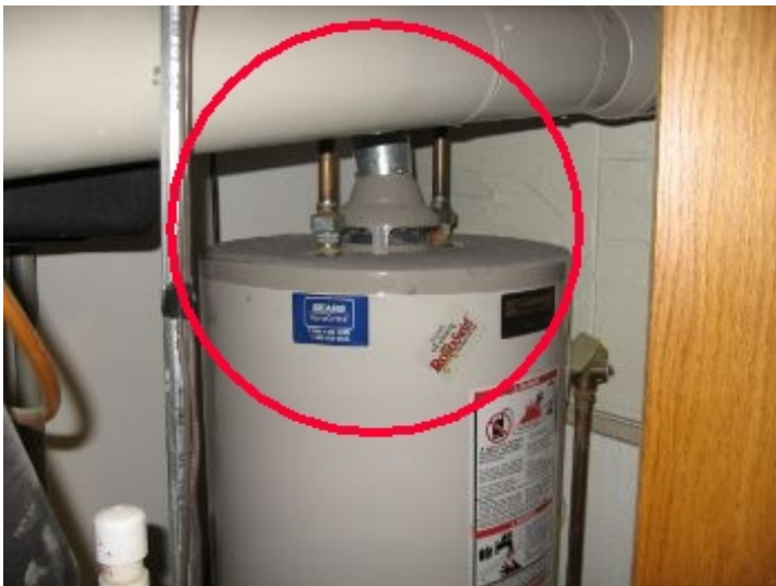
View of water heater venting and water lines
