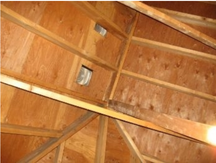
View of upper roof structure (info only)
