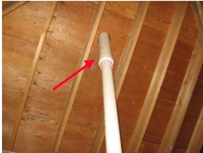
View of plumbing vent roof intersect (info only)
