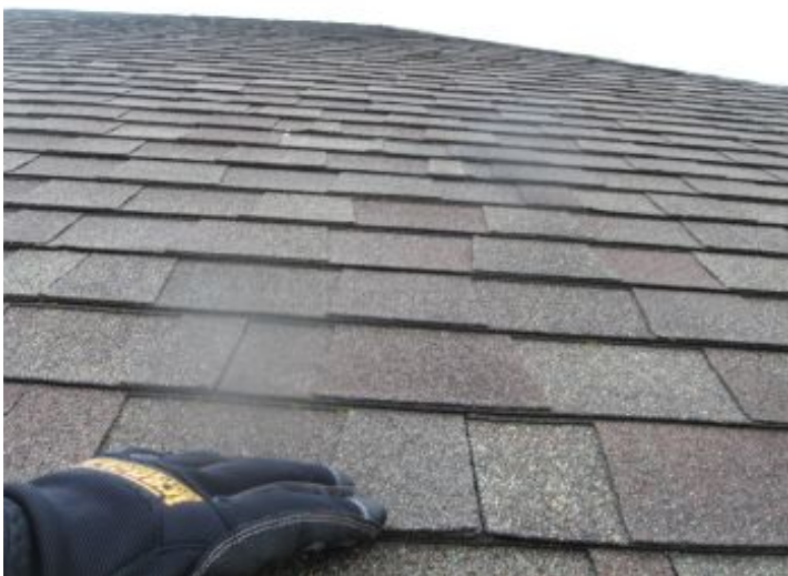
View of overall condition of roof (info only)
